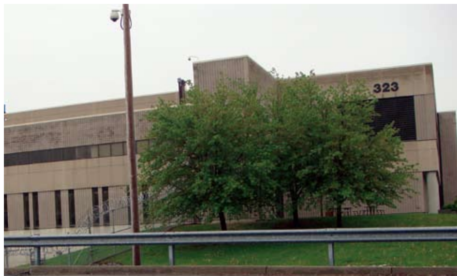
Above: IBM Building 323 East Fishkill, NY, semiconductor plant completed.
